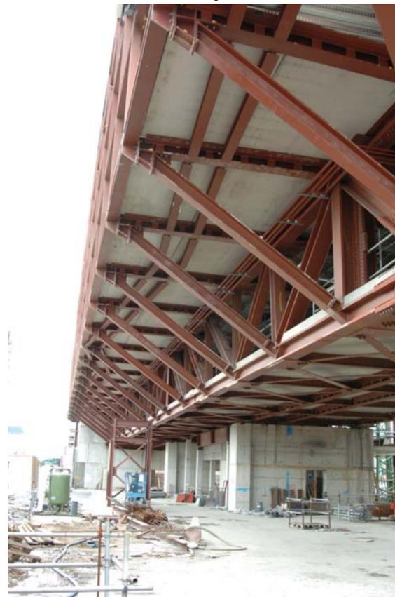
Phased steelwork erection of the upper stories poses further challenges, as the architectural chequerboard pattern design is actually part of the frame, rather than just a style gesture. The steel columns had to be offset relative to the floor below at alternate levels to accommodate the position of the building's glazed panels, and to achieve a thin continuous vertical joint. "Basically the cladding dictates this part of the project," explains Mr. McNelis.
