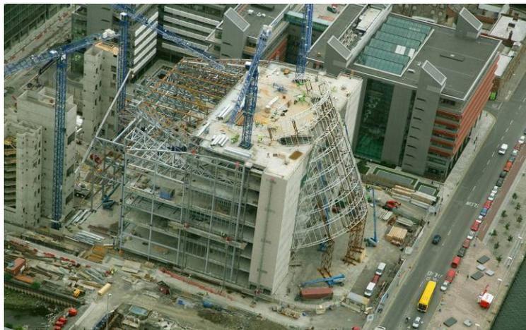
Steel erection began on the south side of the site and has since progressed, in six phases, steadily northwards away from the two southern concrete cores. The structural stability for the building is derived from the two southern RC cores, steel sway frame action of two main frames and also braced frames. The southern RC cores
