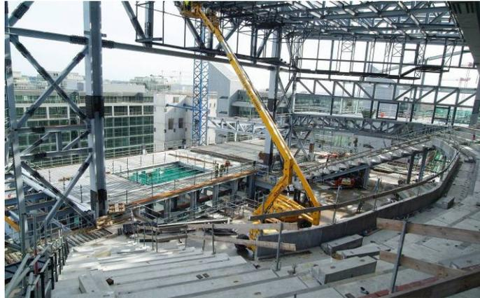
up through the two exposition halls and top out at the roof level of the auditorium. The concrete floor plates utilize composite action metal decking, typically 150mm deep.
