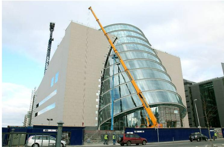
floor to ceiling heights being so high, the perimeter steelwork incorporates secondary 400mm x 200mm and 350mm x 350mm box sections to accept the rail system for the stone cladding.
