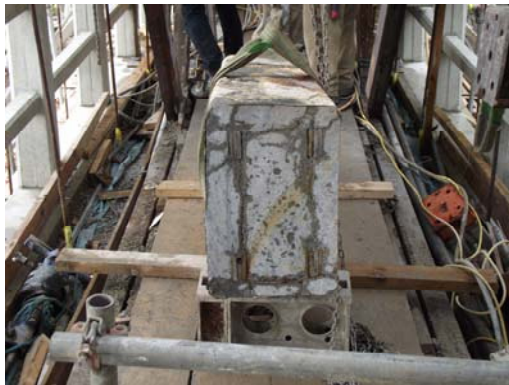
Figure 25: Section of demolished arch rib.
