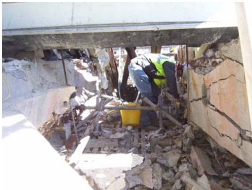
Figure 26: Demolishing the ribs and braces in the back span.
