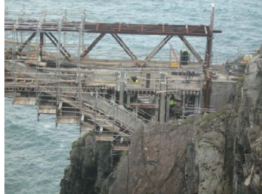
Figure 22: Construction of trestles in back-span
