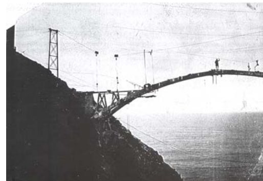
Figure 3: The original bridge under construction
