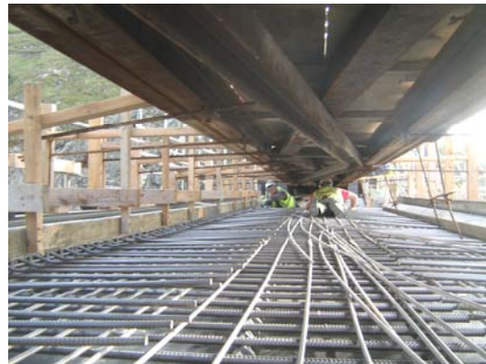
Figure 23: Fixing deck reinforcement in the back-spans
