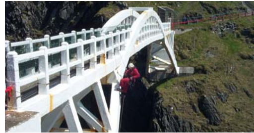
Figure 5: Inspection by roped access in 2002
