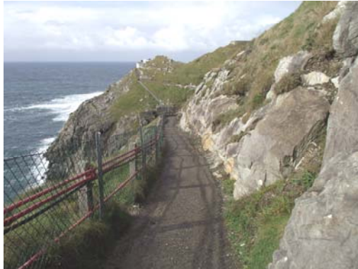
Figure 4: Access to the footbridge
