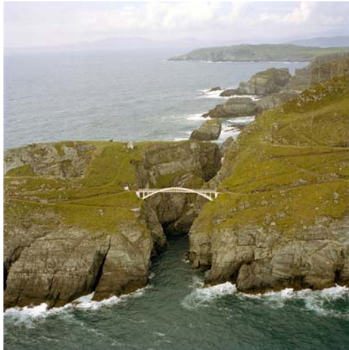
Figure 1: Mizen Head Footbridge (2004)
