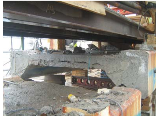
Figure 18: Demolition of the bridge deck by wire saw-cutting.
