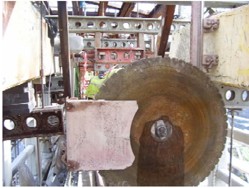
Figure 24: Use of circular saws for demolition.
