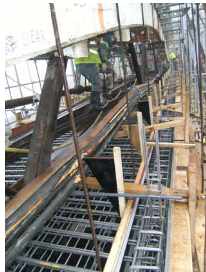
Figure 20: New deck reinforcement
