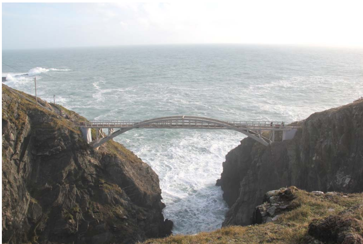
Figure 30: The completed structure
