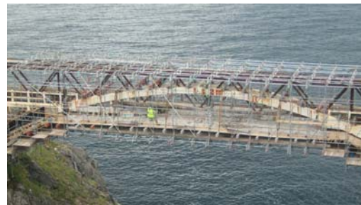
Figure 19: Original deck and hangers removed from the bridge.
