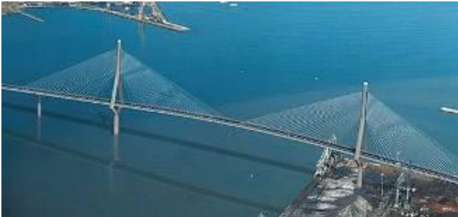
Cadiz Bay Bridge. 560m main span (Spain). Fernandez Casado SL. (To be completed in 2011).
