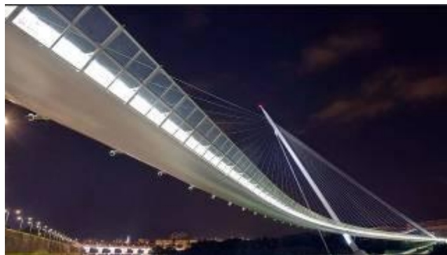
Zaragoza Pedestrian Bridge. 194m main span (Spain). Fernandez Casado SL. (completed in 2009).
